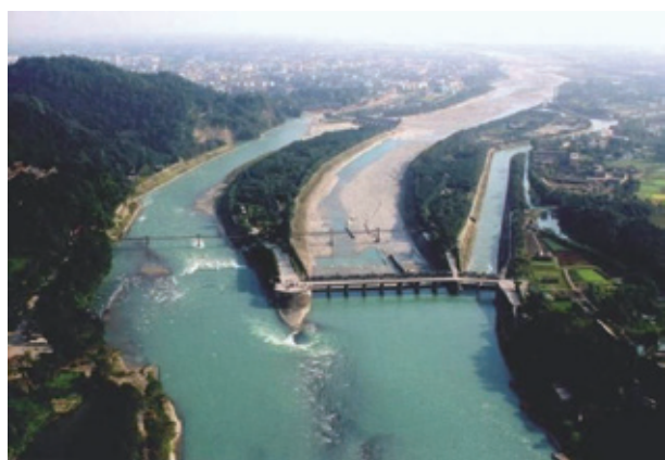
Fig. 5 Dujiangyan water conservancy project 5
