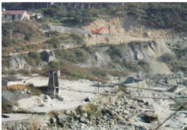
Fig.8 Environment deterioration at Minjiang 10
