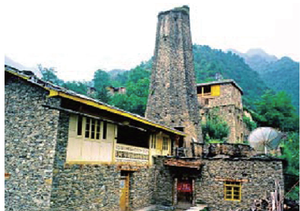
Fig.8 Watchtower residential buildings
