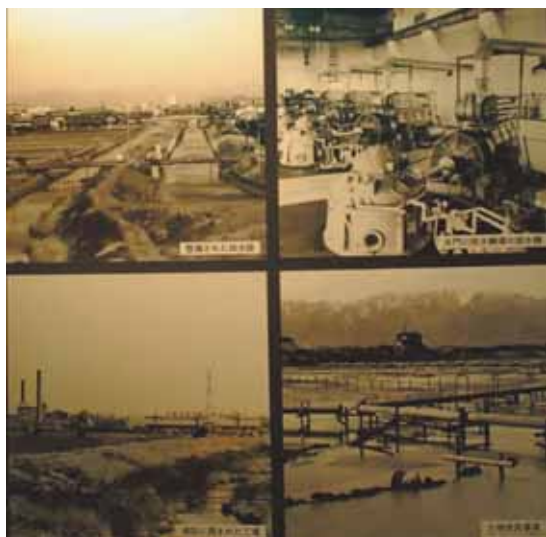
Fig. 6: Left-top: Improved overflow Right-top: Drainer in Watergate River Drain Facility Left-bottom: Factory surrounded by embankment Right-bottom: Land improvement projects (landfill with sand pump) (all are taken by authors)
