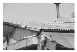
Figure 4. Roof boards including Asbestos
