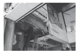
Figure 3. Amosite in the destroyed building
