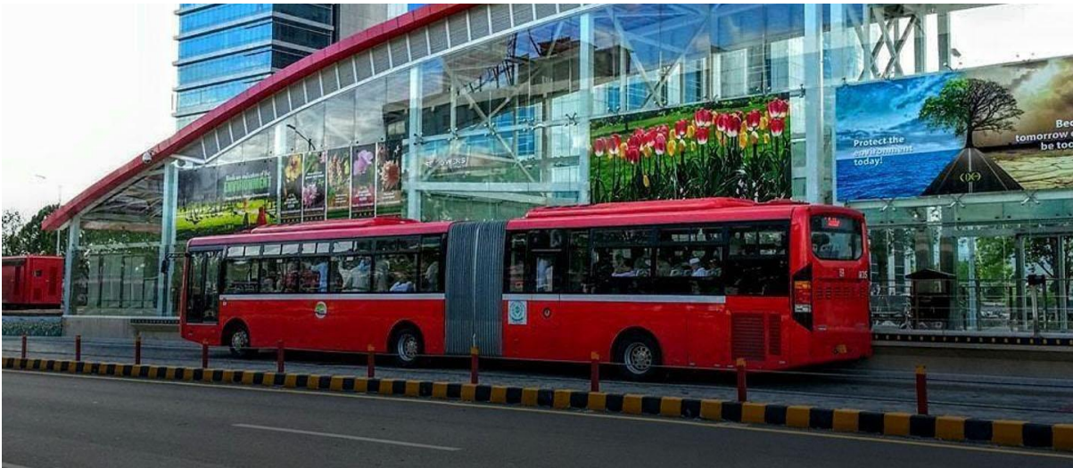
Figure 6 Bus rapid transit in RIMA Source: https://www.zameen.com/
