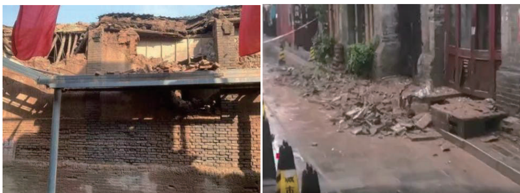
Fig. 3 Damage to buildings and streets in the ancient city 2)
