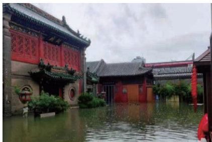
Fig. 2 Water in the Hall
