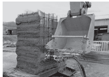
写真 21 On-Site Shot Printer
