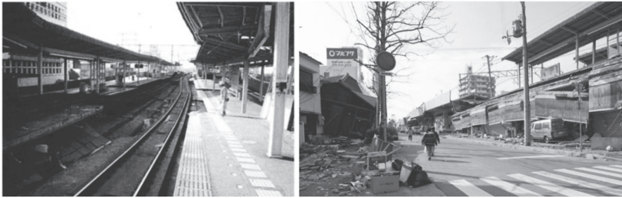
Fig.1. Rokkomichi Station (JR-West)
