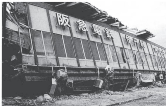
Fig.3. Itami Station (Hankyu Railway)
