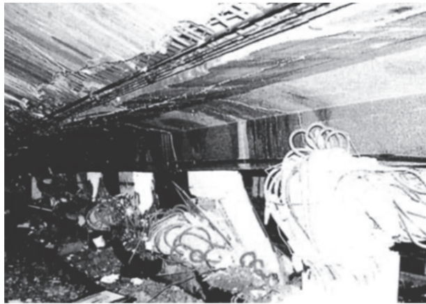
Fig.5. Daikai Station (Kobe Rapid Transit Railway)
