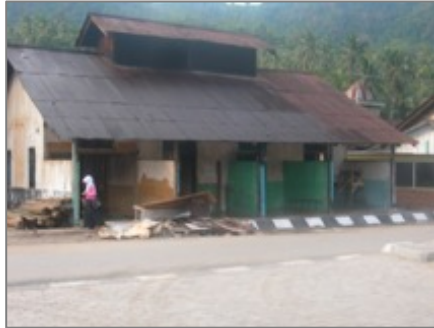
Ex-miner housing before revitalization project
