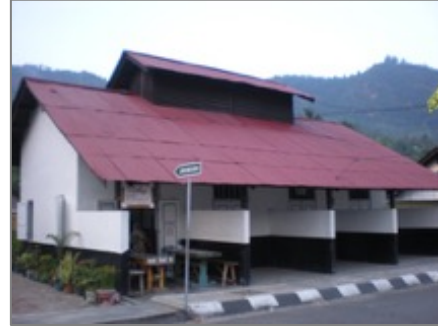
Ex-miner housing after revitalization project
