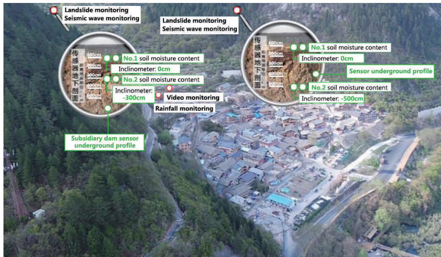
Figure 4 Location of seismic sensor and acquisition instrument
