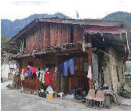
Fig. 12 Few Structures Damaged
