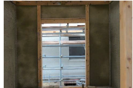
(c) 桁行土壁
