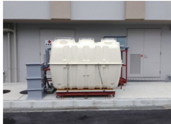
Photo 2. Installed Johkasou
