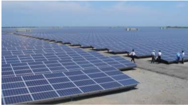
Fig. 4 JGC Mega solar system with 26MW at Oita industrial zone (Author shot)
