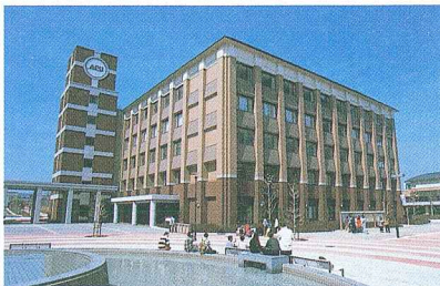
Building A — Administration A棟 (本部棟)
