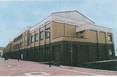
Building H — Graduate School H棟 (大学院棟)
