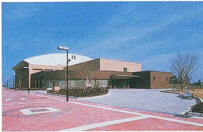
Building G — Gymnasium G棟 (体育館)
