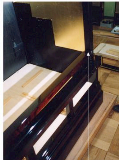
upper chuuji attached to groove B (see kumi photo 09)
