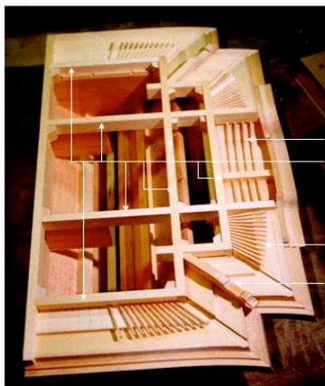
Kuuden photo 26: beams, a few taruki in position
