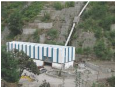
(b) 5 MW Andhra-II Small Hydro Power Project in Himachal Pradesh
