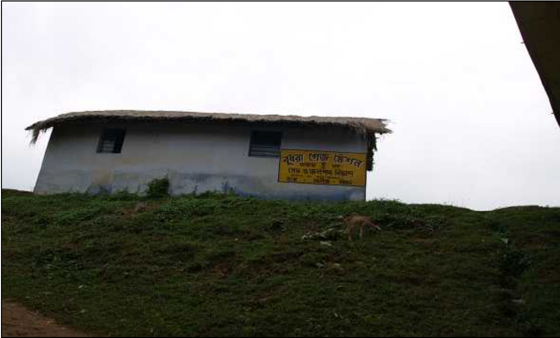
The Budhra gauge station near Bolpur
