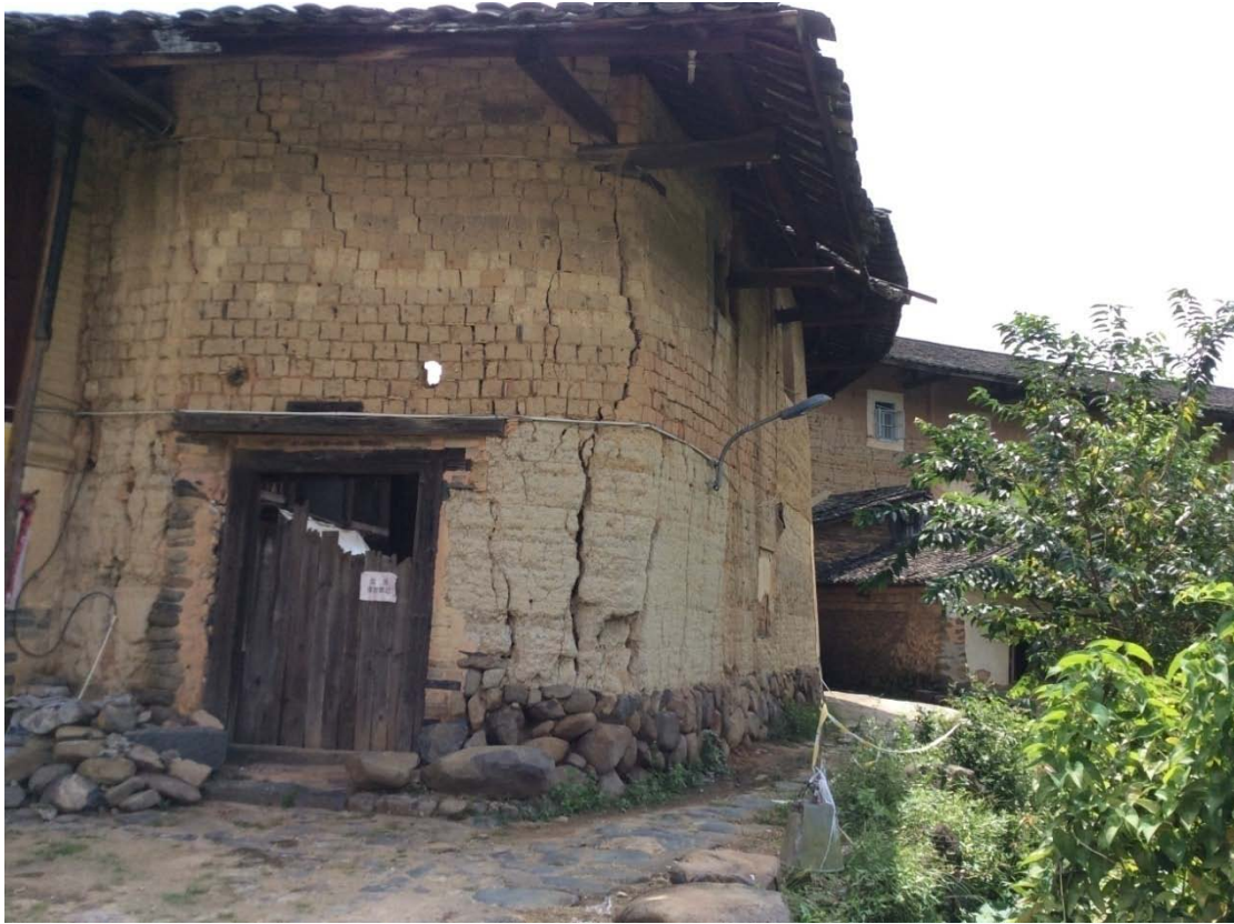
Figure 5.6 The exterior of a tulou in danger Source: taken by the author (September 2015).
