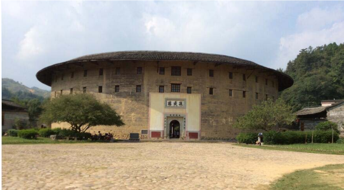
Figure 5.2 The exterior of Zhencheng Lou
