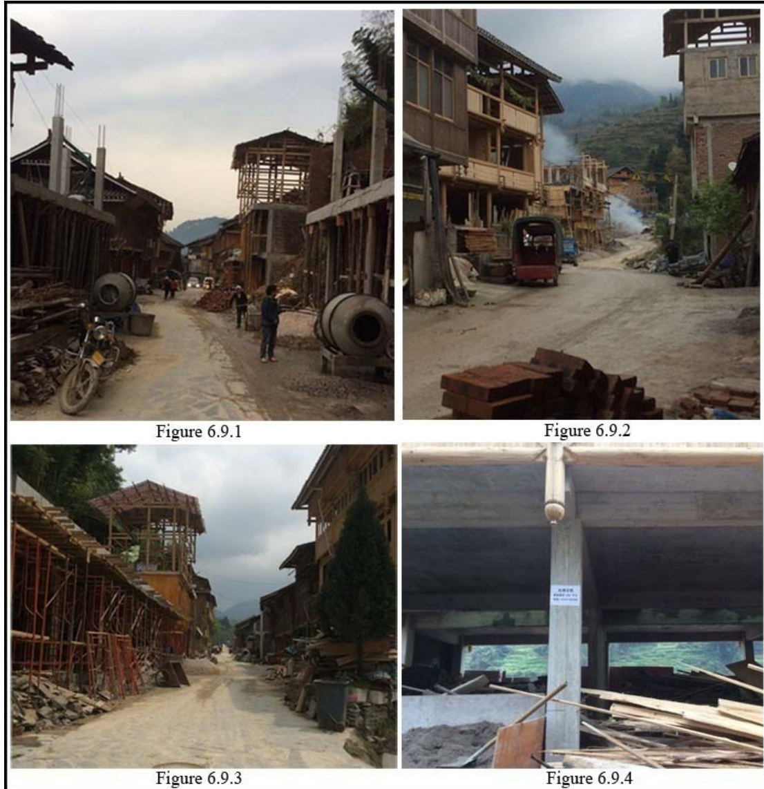
Figure 6.9 Houses being built in Zhaoxing Source: taken by the author (March-April 2016).
