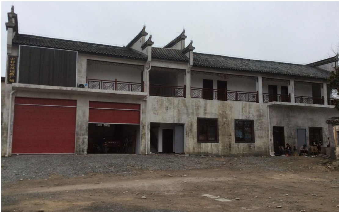
Figure 6.6 A two-storey concrete building built by the township government
