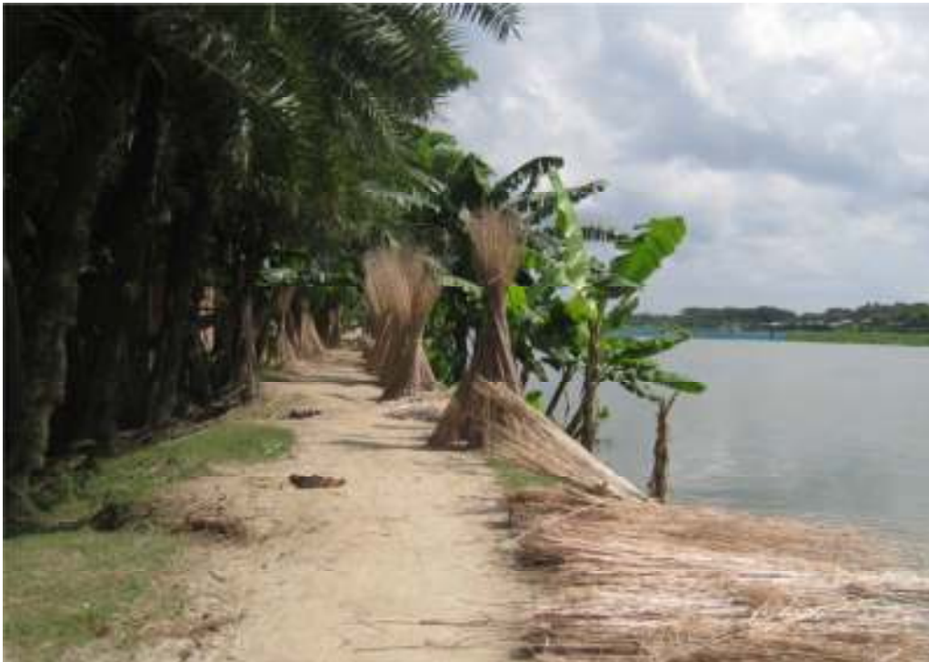
Image 5.5. The Embankment in Chandra Village to Protect Floodwater Intrusion
