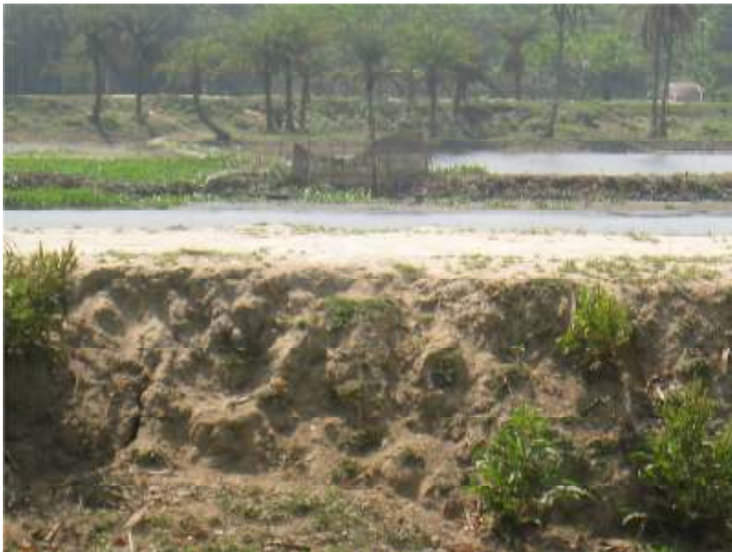
Image 5.5 Embankment ( Kacha road) in Chandra Village
