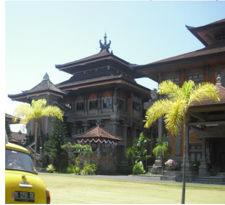
Figure 2.2b Common urban style building in Bali
