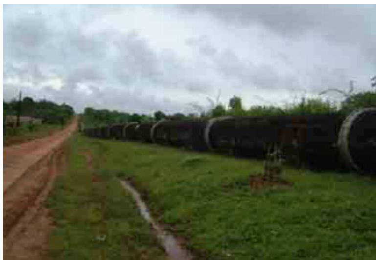
Transmission Main Pipe in City Water Supply System
