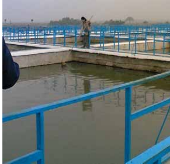
Cleaning Floating Material from Water Treatment Plant by Manual Practice in City Water Supply Project
