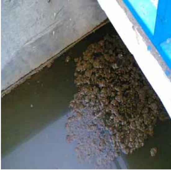
Cleaning Floating Material from Water Treatment Plant by Manual Practice in City Water Supply Project
