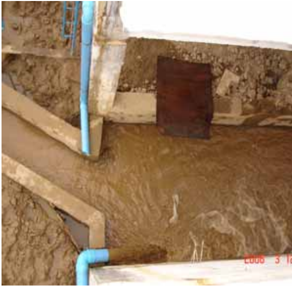
Sludge Disposing Practice from New Water Treatment Plant (This Water Drainage to Agricultural Paddy Field)
