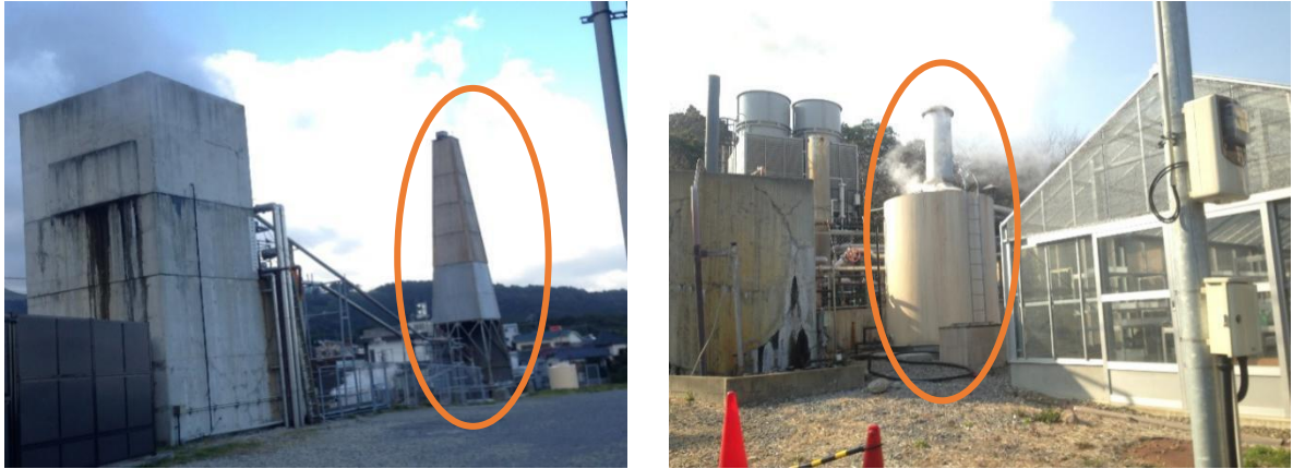
Figure 7 Cooling towers for hot spring water in Beppu
