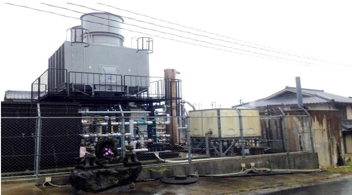
Image 3: Binary hot spring geothermal facility built alongside a conventional hot spring extraction, cooling and distribution unit at Miyamae onsen in Kanawa district of Beppu city Source: Author
