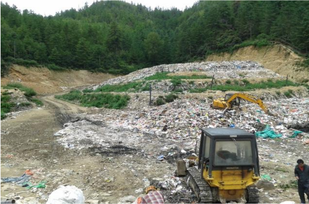
Figure 6. 1: Memeylakha Landfill, Thimphu City (site visited)
