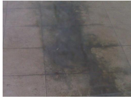
Picture 5.4. Leakage in dwelling units
