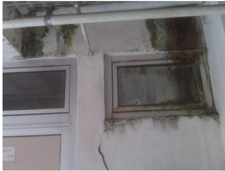
Picture 5.4. Leakage in dwelling units
