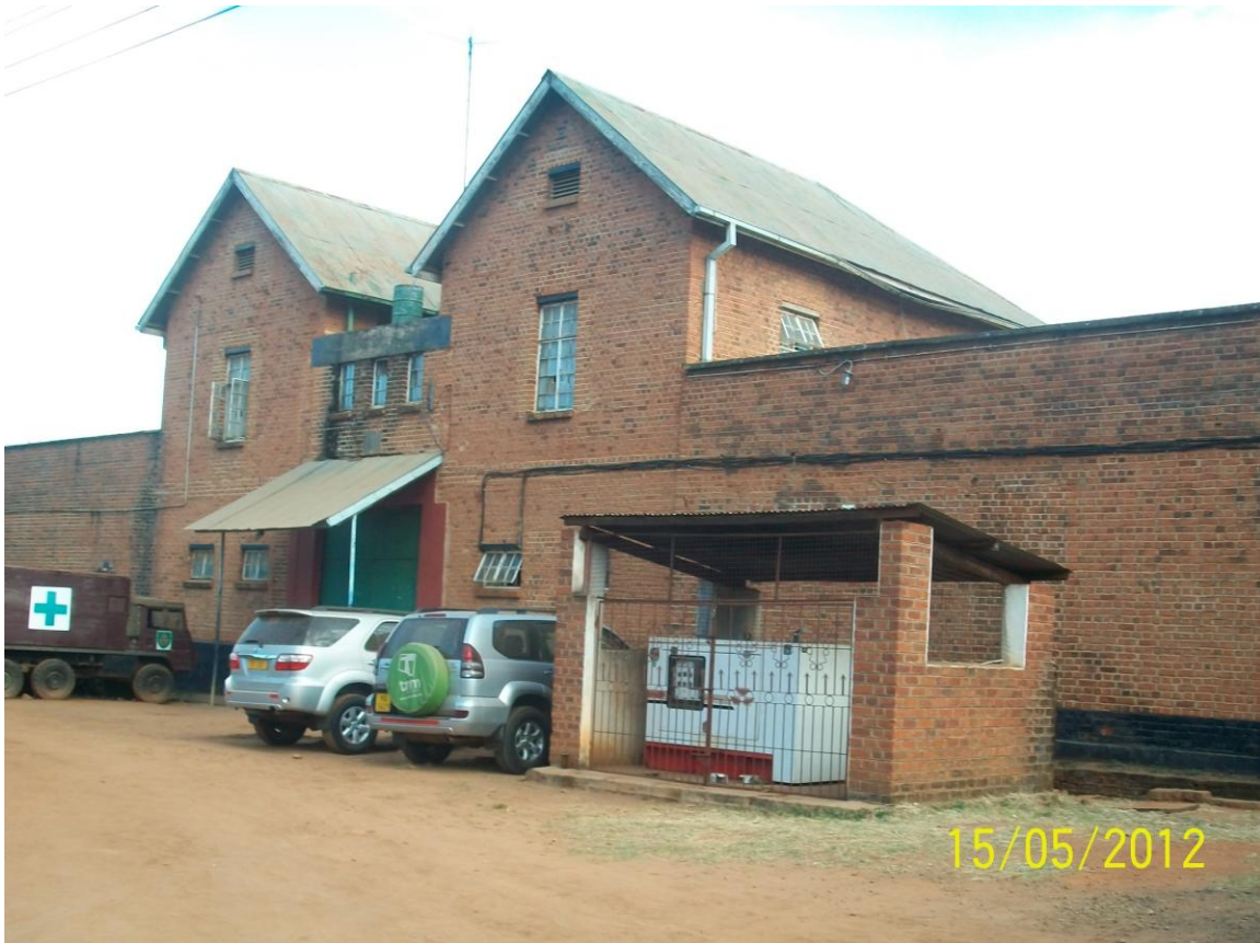
Figure 2.1a: Part of the perimeter brick wall fence measuring 12 meters around Zomba central prison
