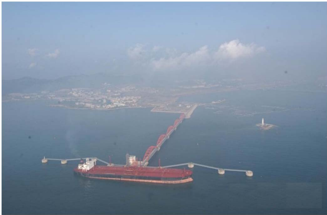
Figure 4.6 Nianyu Bay Port Area
