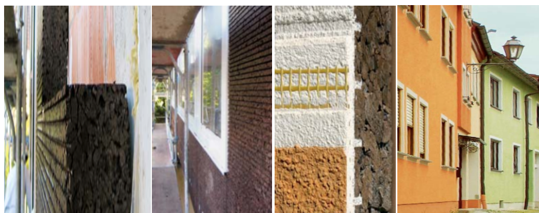
Figure 4.9 Four views of Bio-HAGA Korit insulation installation steps to completion
