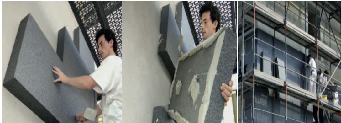
Figure 4.1 Three views of BASF Neopor insulation being installed
