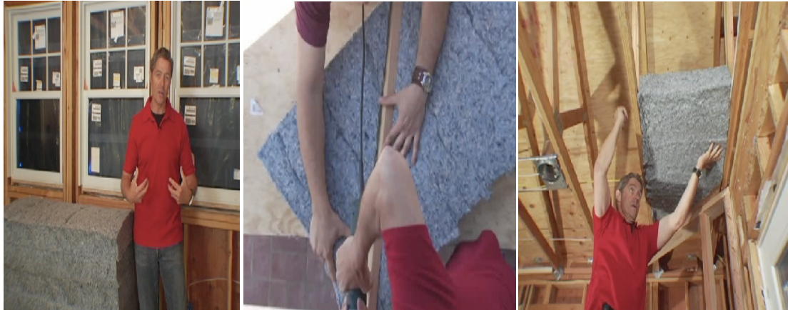
Figure. 4.10 Three views of Bonded Logic Inc. UltraTouch insulation being installed
