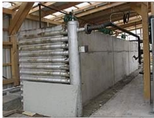
Figure 3.4.6 Concrete thermal storage 14
