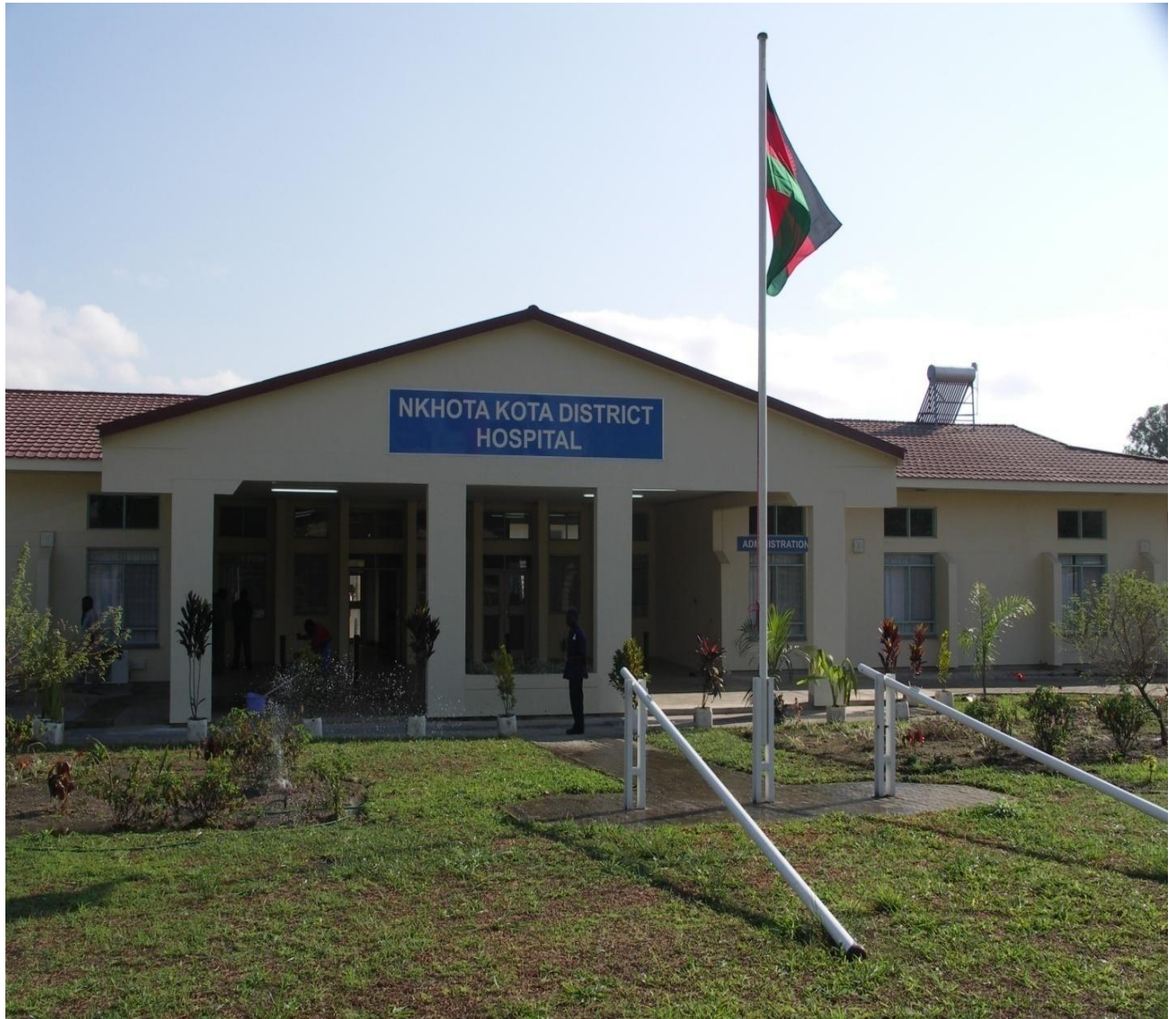
Figure 4.1: The new Nkhotakota District Hospital
