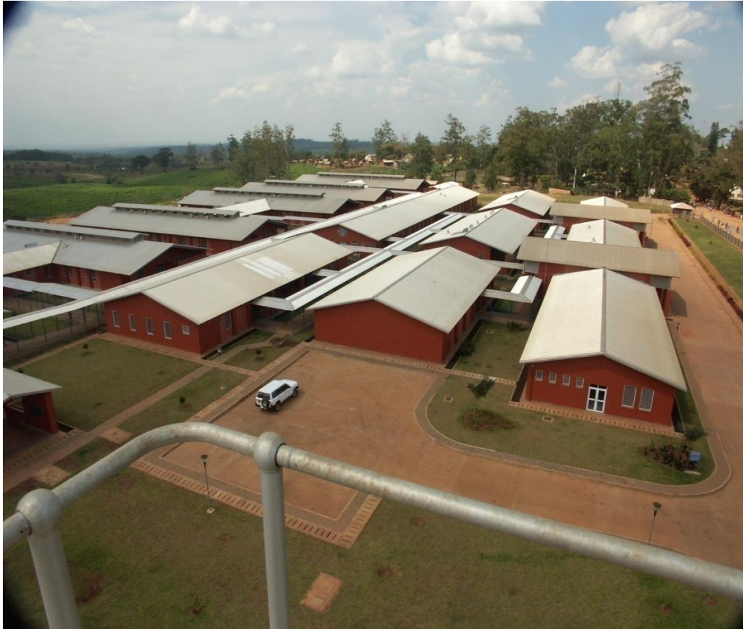
Figure 4.5: The new Thyolo District Hospital (Aerial View)
