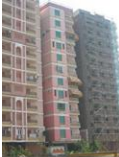
Figure 2.4 - Picture showing blocked windows and different finishes for apartments in the same building
