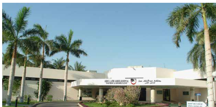
Figure 4.7 - The building D
