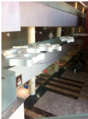
Figure 4.10 - The Entrance Ceiling Height
