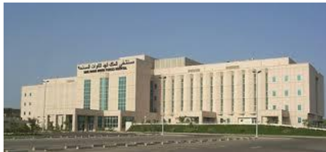
Figure 4.6 - Building C Facade
