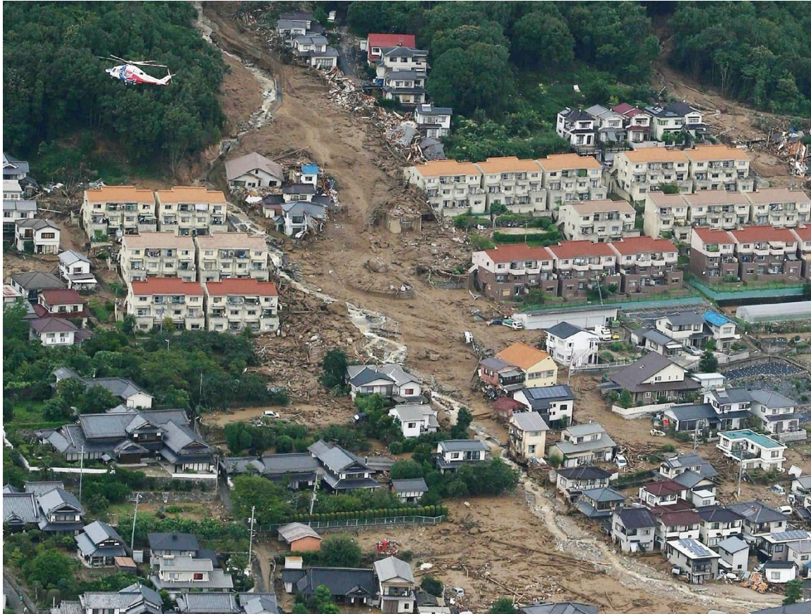
Figure 1.2: Landslide in Hiroshima, Japan 2014 (source from http://www.thetimes.co.uk )
