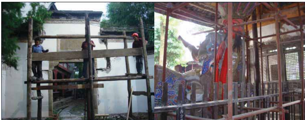
Fig.5 Temporary reinforcement of historic buildings
