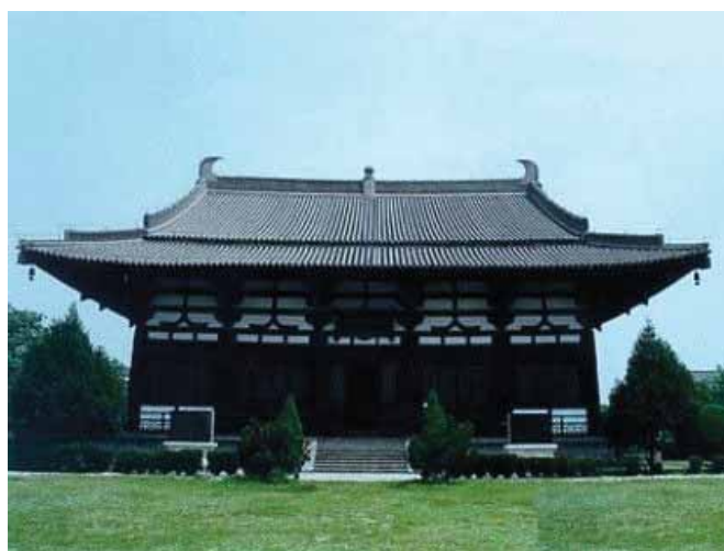
Fig.2 Damaged historic building in national cultural heritage
