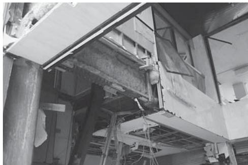
**Figure 3. Amosite in the destroyed building**
