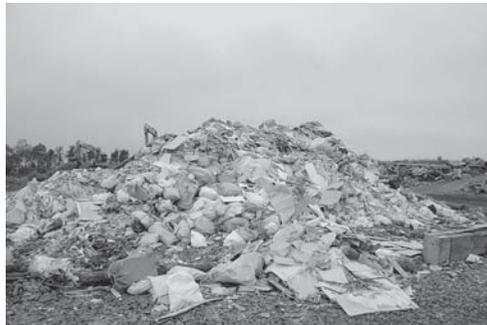
**Figure 5. The boards including Asbestos in the stockyards of rubble**
