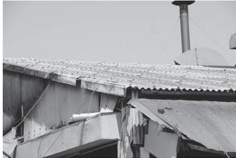
**Figure 4. Roof boards including Asbestos**
