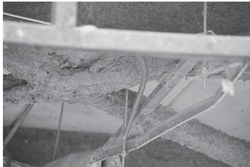
**Figure 2. Crocidolite in the destroyed building**
